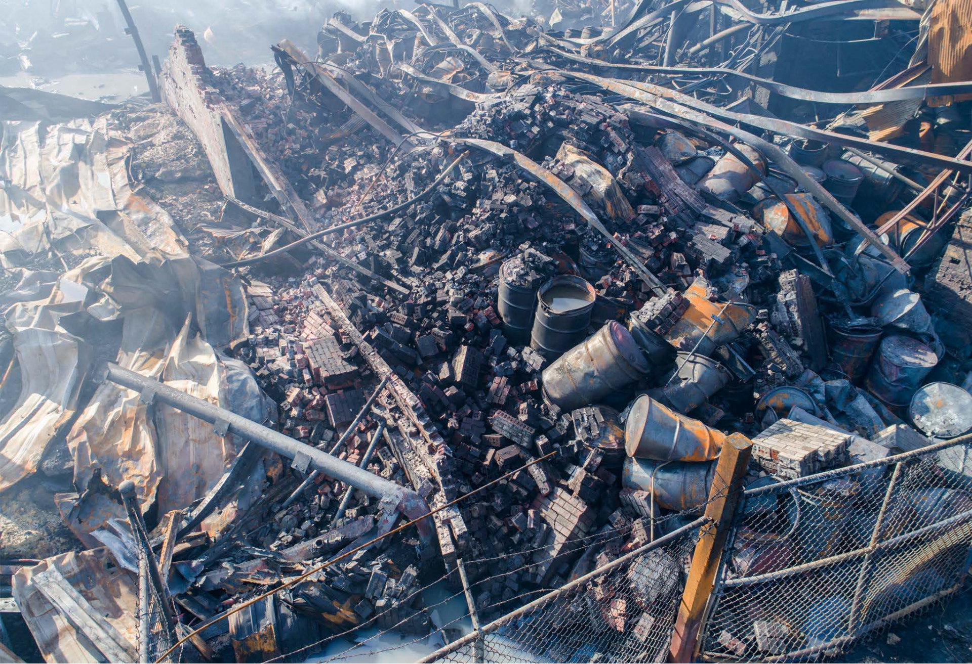
After the Fire – Drums and Debris
