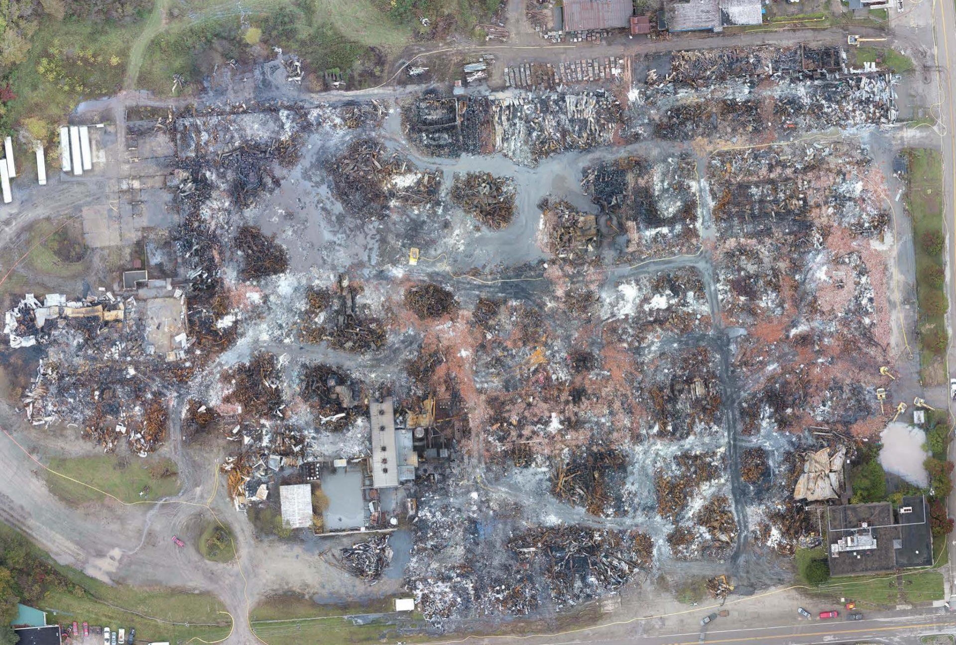
Building Footprint after the Fire
