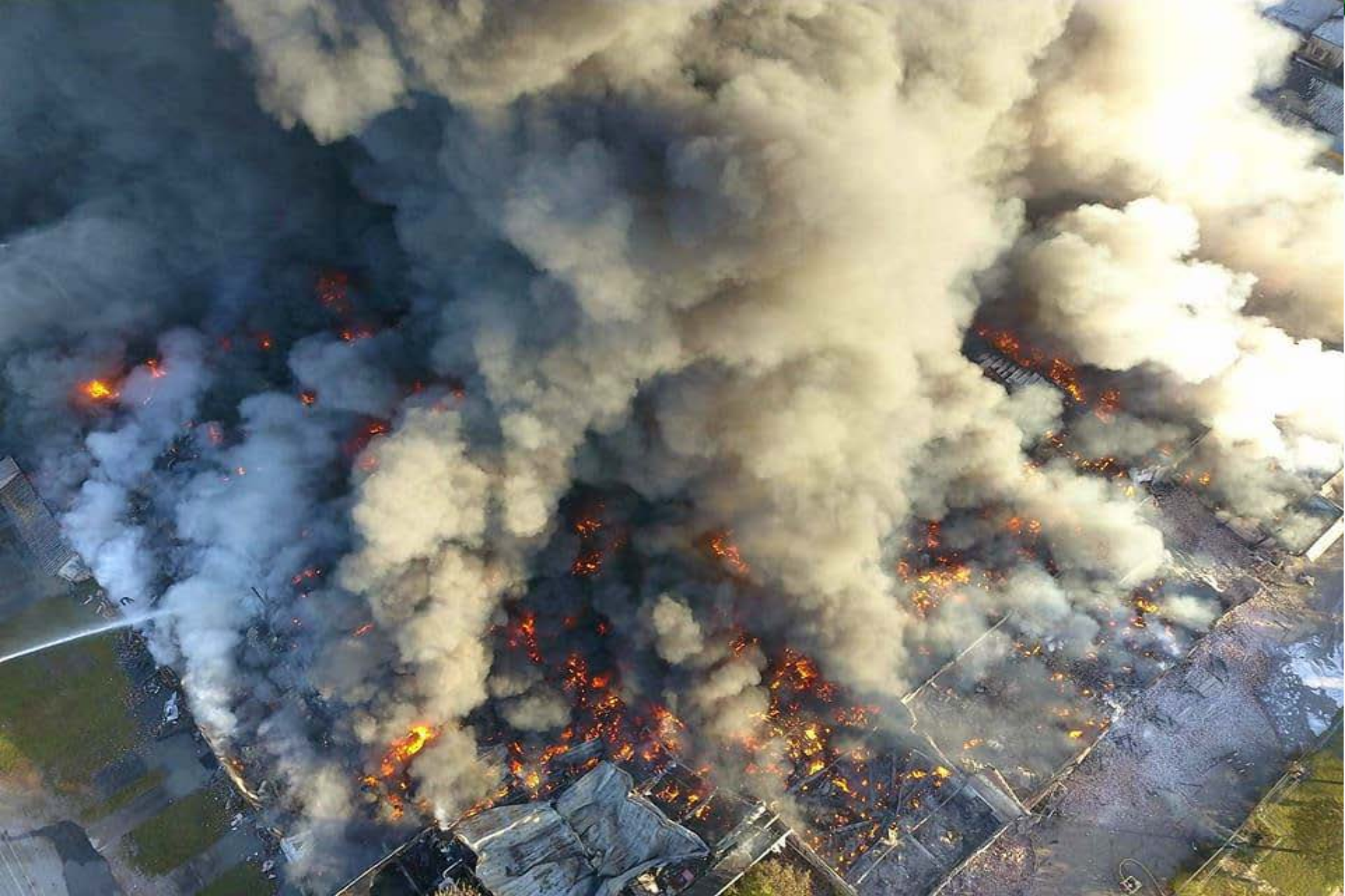
Day 2 Fire Fighting - Entire Building Consumed
