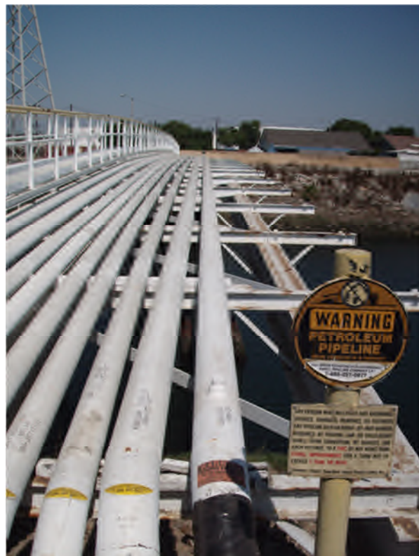
Figure 2- Pipes over the Dominguez Channel
