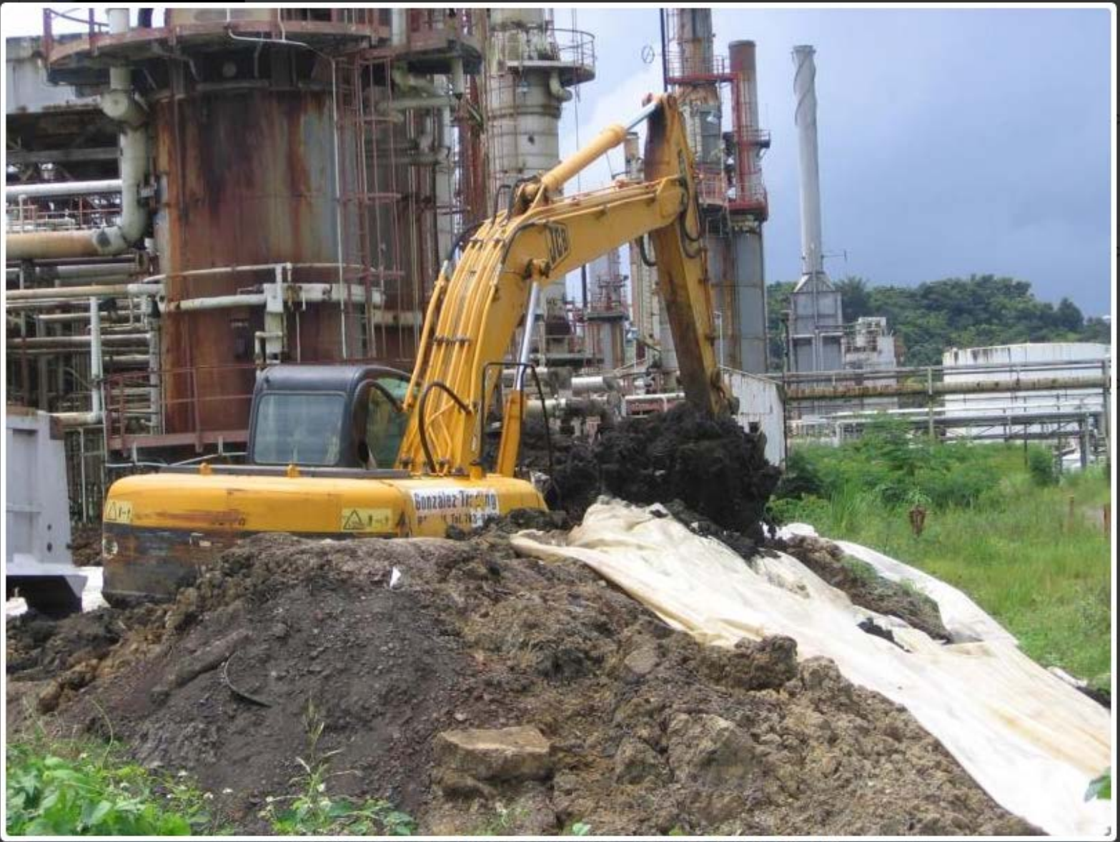
Loading oil contaminated soil
