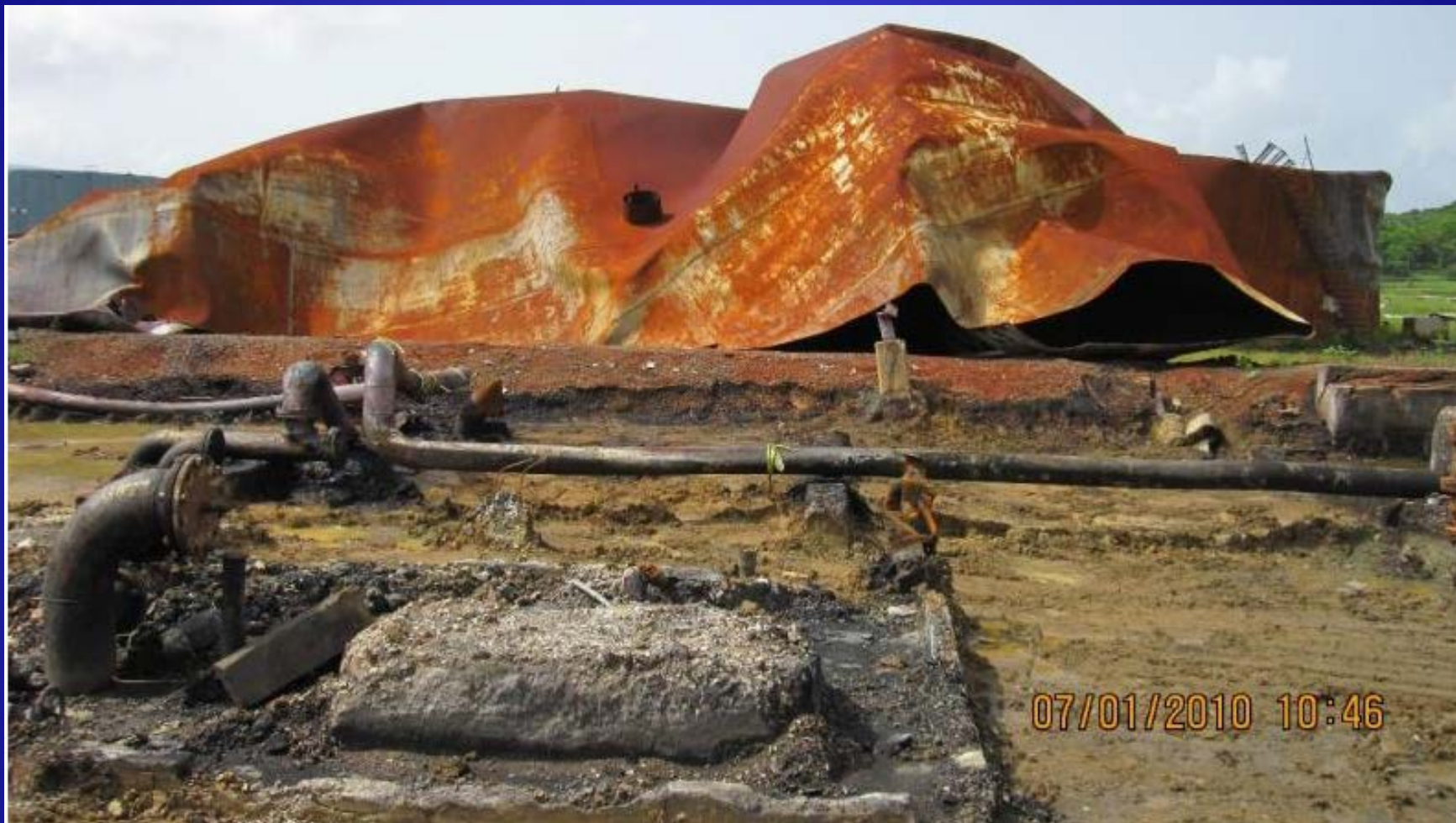
Avenue D after soil/line removal. Tank 503 lid in background
