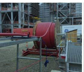
Pulling 15,000 Volt Cable to Substation
