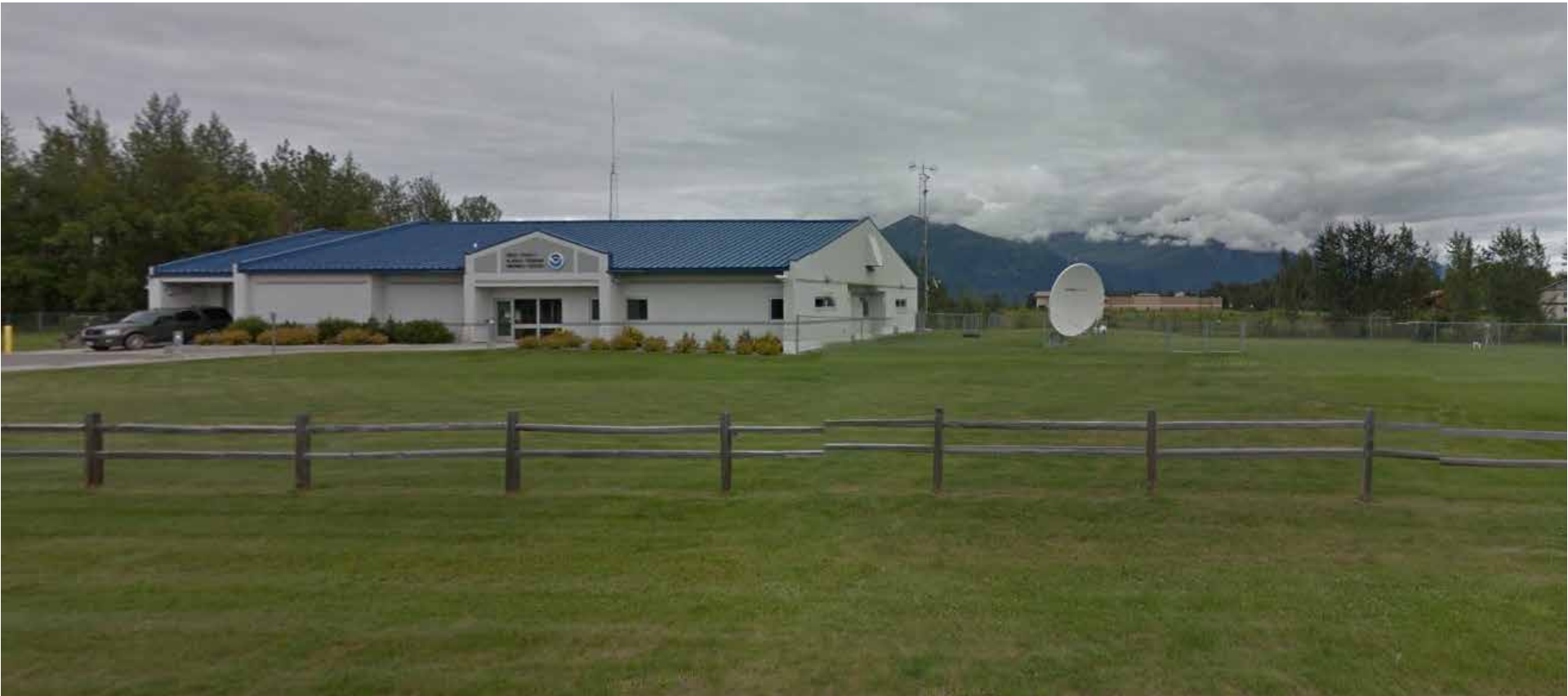
National Tsunami Warning Center, Palmer, Alaska
