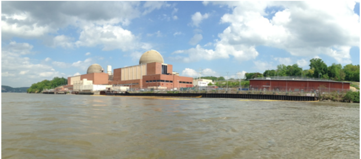
Harbor boom deployed within the Hudson River at Indian Point Nuclear Plant, Buchanan, New York.
