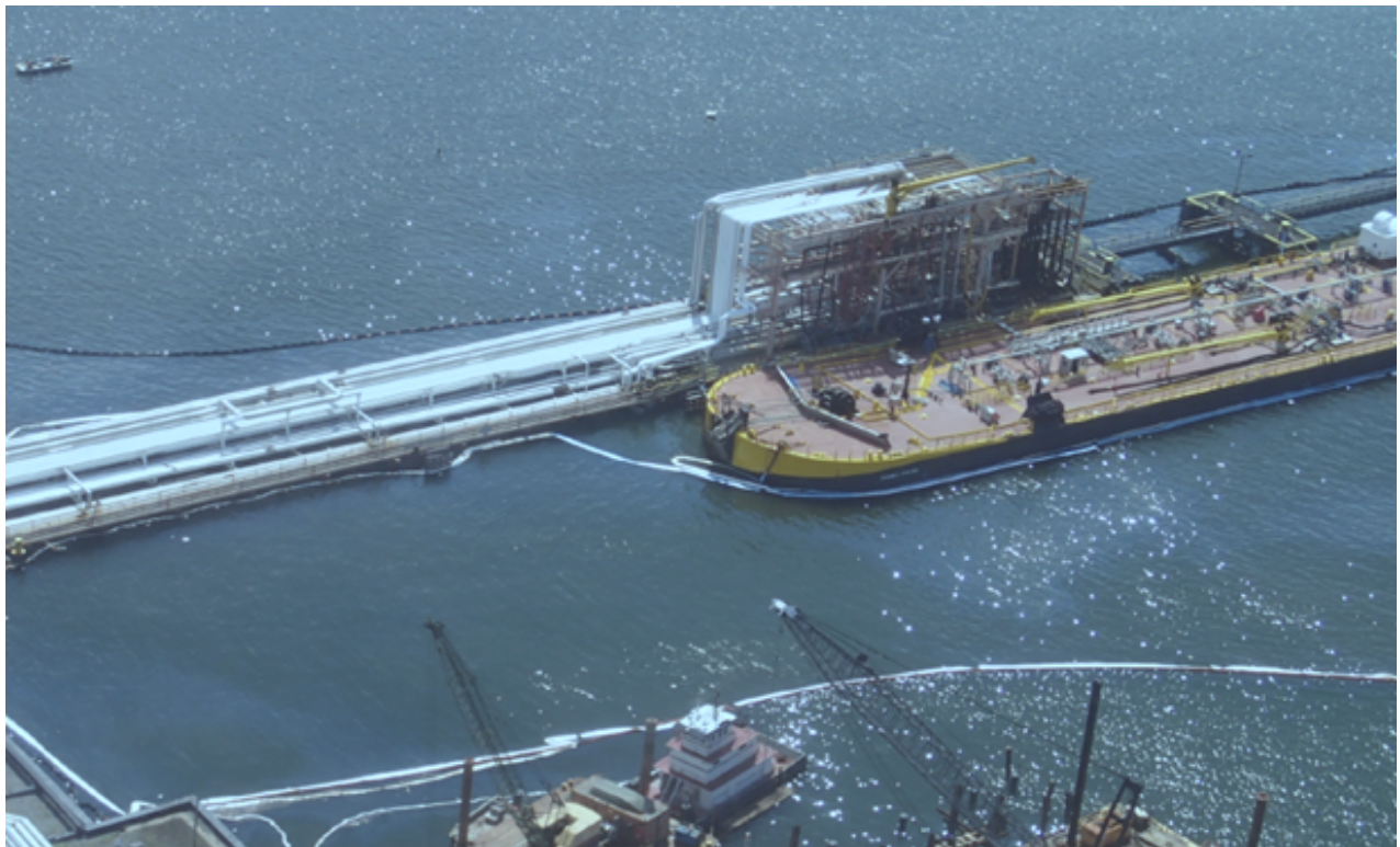
Pier Alpha damaged by Tug PETER F. GELLATLY and release of 400-800 gal No. 6 Fuel Oil.
