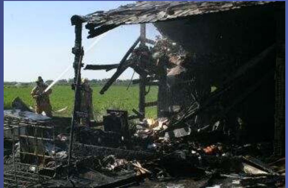
Fire at biodiesel plant in Canby, OR (06/24/2006) Source of the blaze was the biodiesel. Methanol tanks were unaffected.
